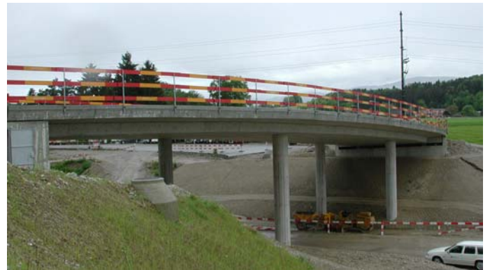
Figure 1. View of the bridge.
