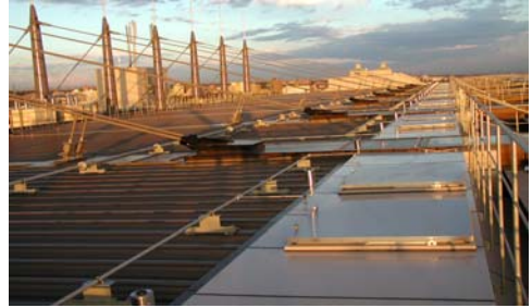
Figure 1(b) The roof of the Stadium
