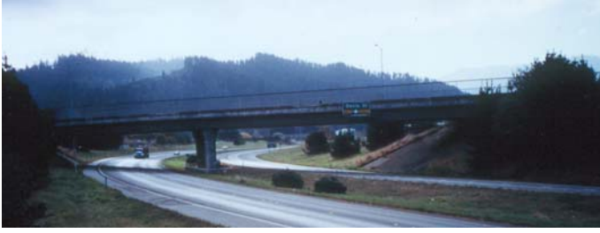
Figure 1. North side view of Painter Street Overpass.
