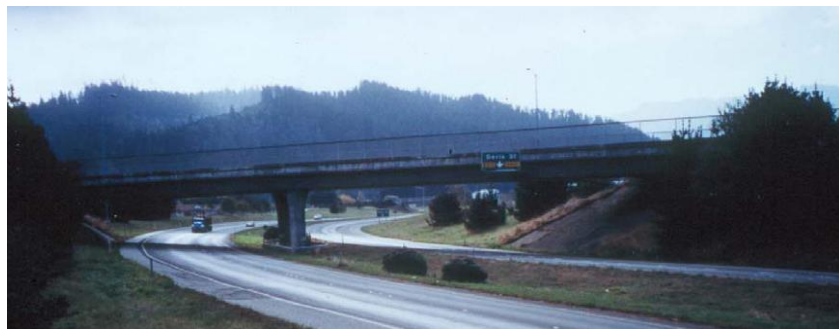
Figure 1: Painter Street Overpass Bridge.
