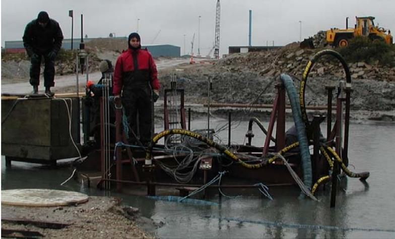
Figure 6. The 4x4 meter test bucket successfully installed.
